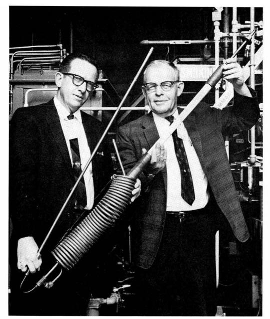
REPAIR rather than replacement of three palladium-silver diffusion cells similar to the one displayed by Dave Watt (left) and E. R. Wood saved Sandia Laboratories \$18,000 and 13 weeks of time.
